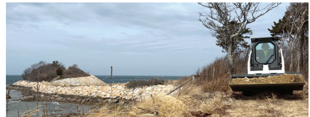
Subcontractor Rich Clements shuttling a load of cobble mix from the staging area to the outer harbor bank erosion project site for the 2026 supplementation
