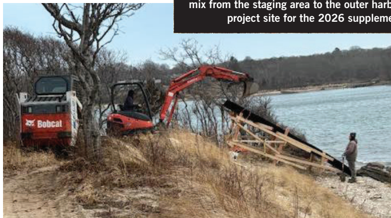
Bill Armstrong using a long reach mini-excavator to load cobble into a delivery chute mounted on a movable trestle; Fritz Kaufmann on the cobble berm standing by to spread the cobble.
