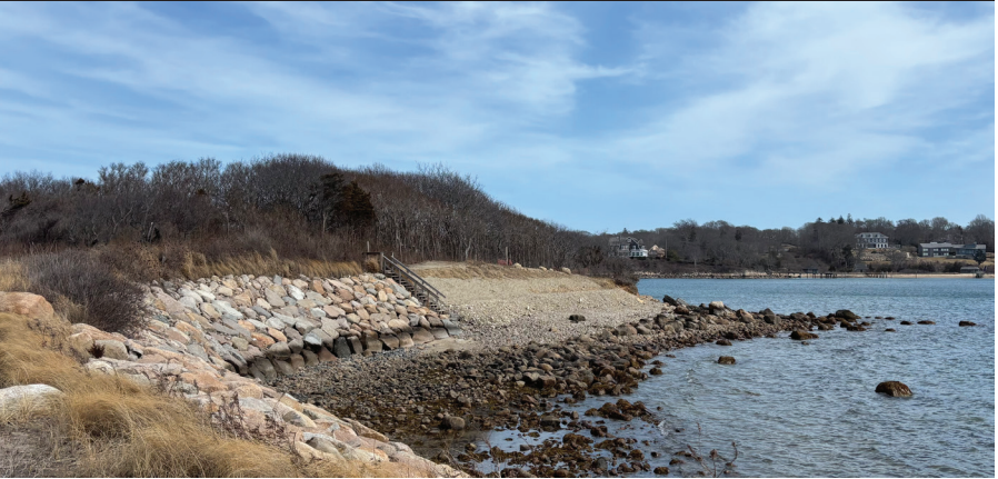
The recent work on the outer harbor bank (to the right of the wooden staircase) has reinforced the bank with an array of anchored coir logs and protected that array with a mobile berm of wave-dispersing rocks and gravel at the base of the bank.
