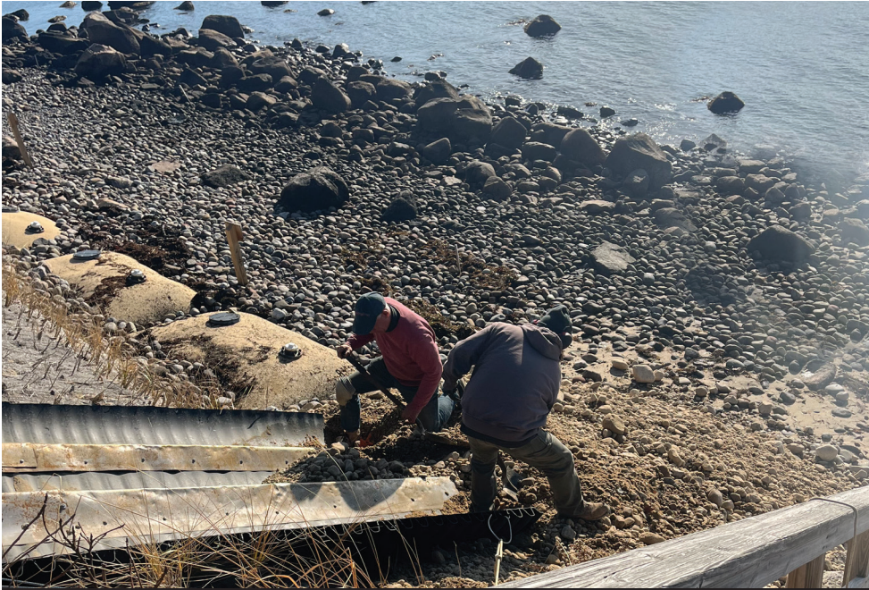
Bill Armstrong and Fritz Kaufmann use custom-made chutes to deliver additional cobble mix to the inner harbor bank next to the wooden stairs.
